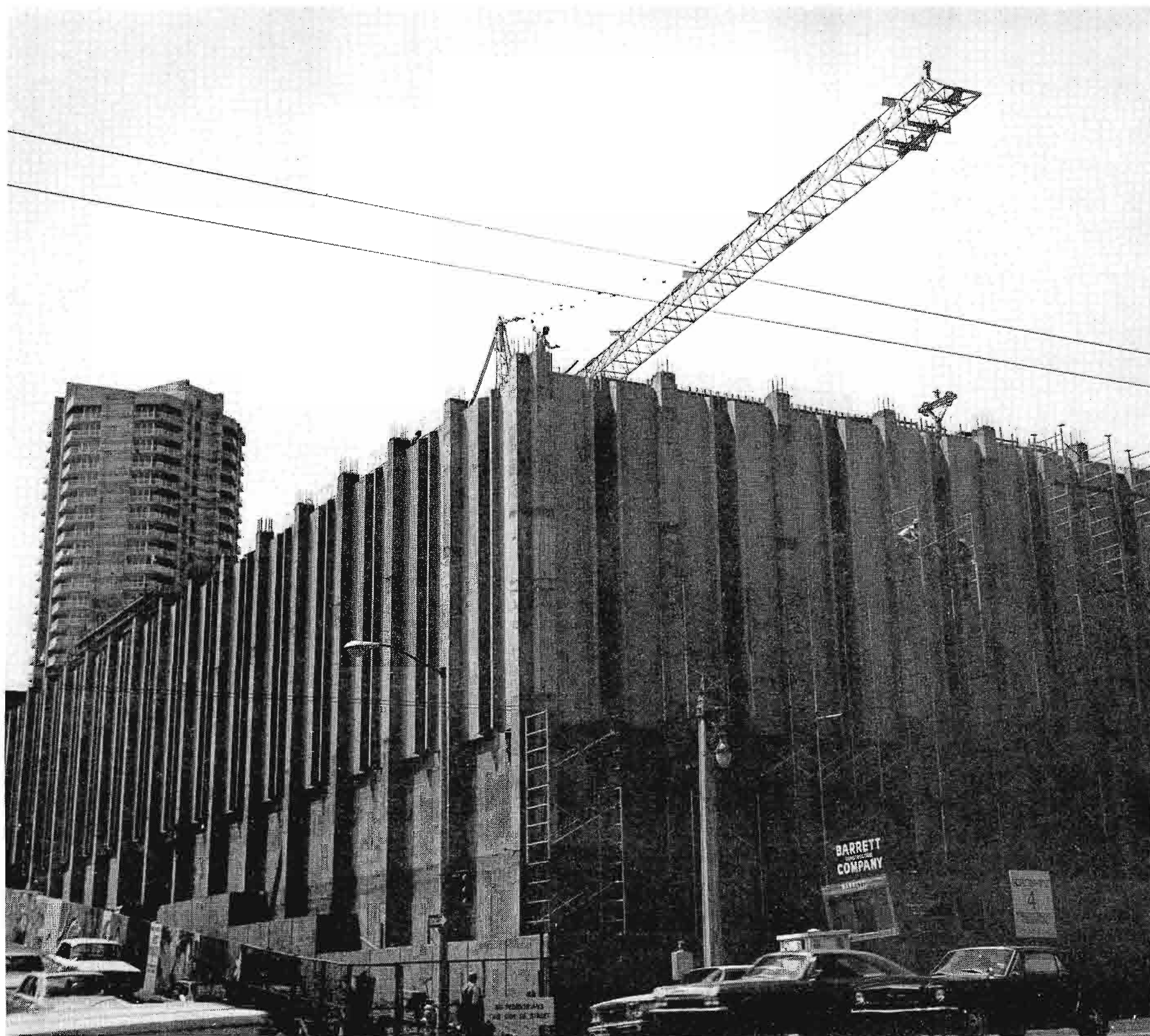
FIG. 21. This shows the KRON-TV building during the construction phase. The nature of the location can be seen by noting the sharp incline of the street. The front entrance is at first-floor level. An entrance halfway back along the side is at second-floor level. An entrance at the rear is at third-floor level.
